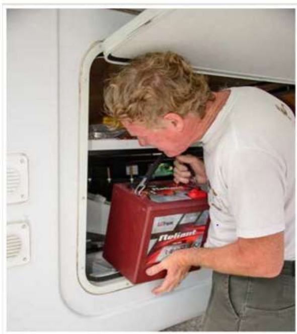
Mark installs the new Reliant batteries in the old plastic battery boxes
